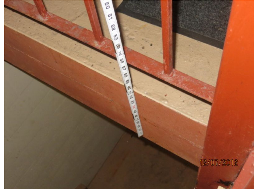
Reinforced Concrete Roof Deck
